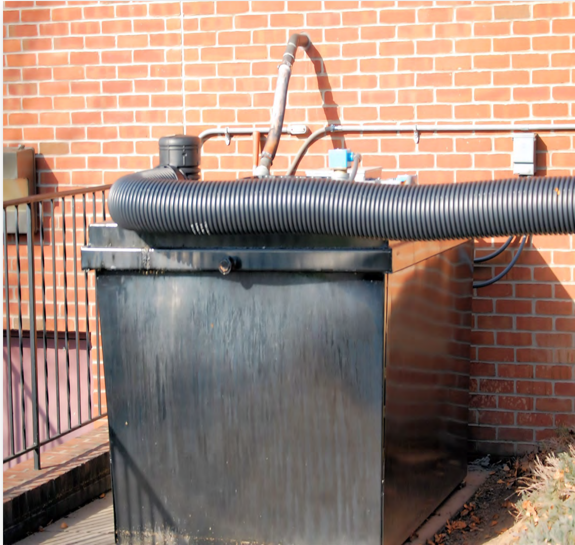
200gl transfer tank (original purpose was grease collection)
